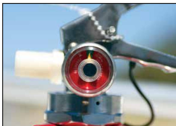
Check the gauge on extinguishers regularly to ensure it's serviceable.
